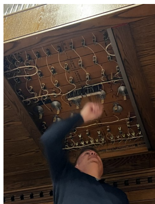
Peder working on organ connections in pipe chamber.
